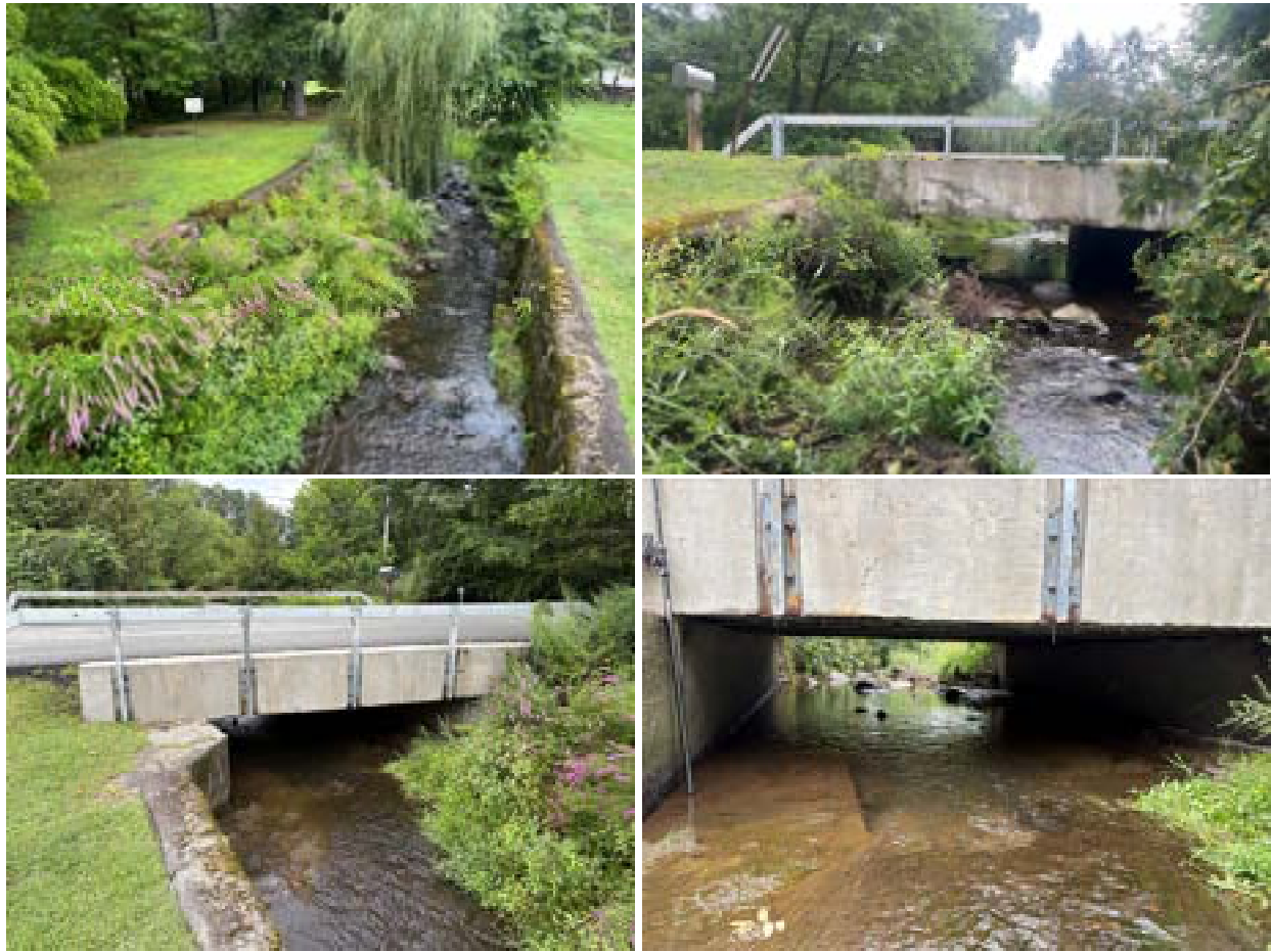
Figure 3. Philips Brook at the Avery Road stream crossing. Clockwise from upper left: Looking upstream from Avery Road at the vertical walls, some sediment accumulation and vegetation growing in the walls; looking upstream at the Avery Road crossing; looking downstream under the Avery Road crossing, noting the concrete walls and concrete footings sticking out into the stream; and looking downstream at the Avery Road crossing, noting the vertical walls and degrading concrete apron upstream of the crossing.
