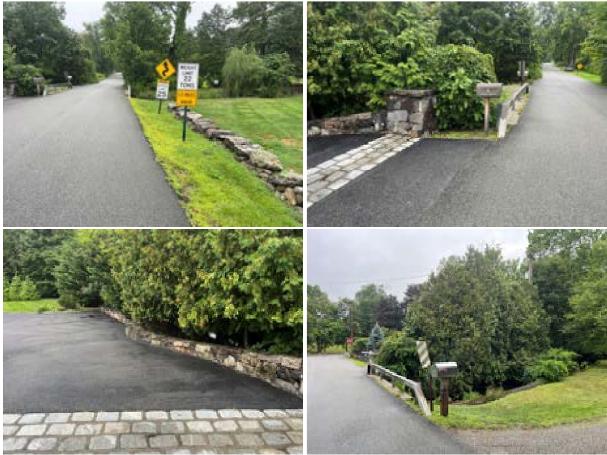
Figure 4. Infrastructure on, and adjacent to, the Avery Road crossing. Clockwise from upper left: looking north, noting street signs and guardrails; looking north on the downstream end of the crossing, noting mailboxes and guardrail; looking south on the downstream end of the crossing, noting mailboxes and guardrail; looking west along the driveway, noting the stone wall separating the driveway from the stream channel.
