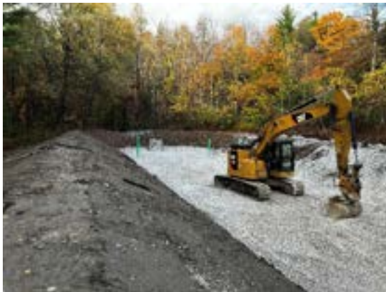
Photo 1: Gravel wetland under construction in October 2025
