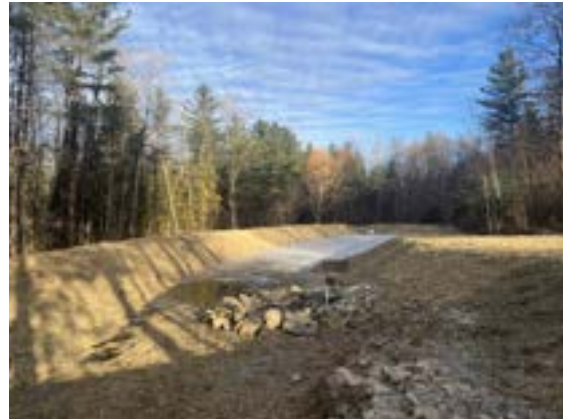
Photo 2: Completed and winterized gravel wetland in December 2025.
