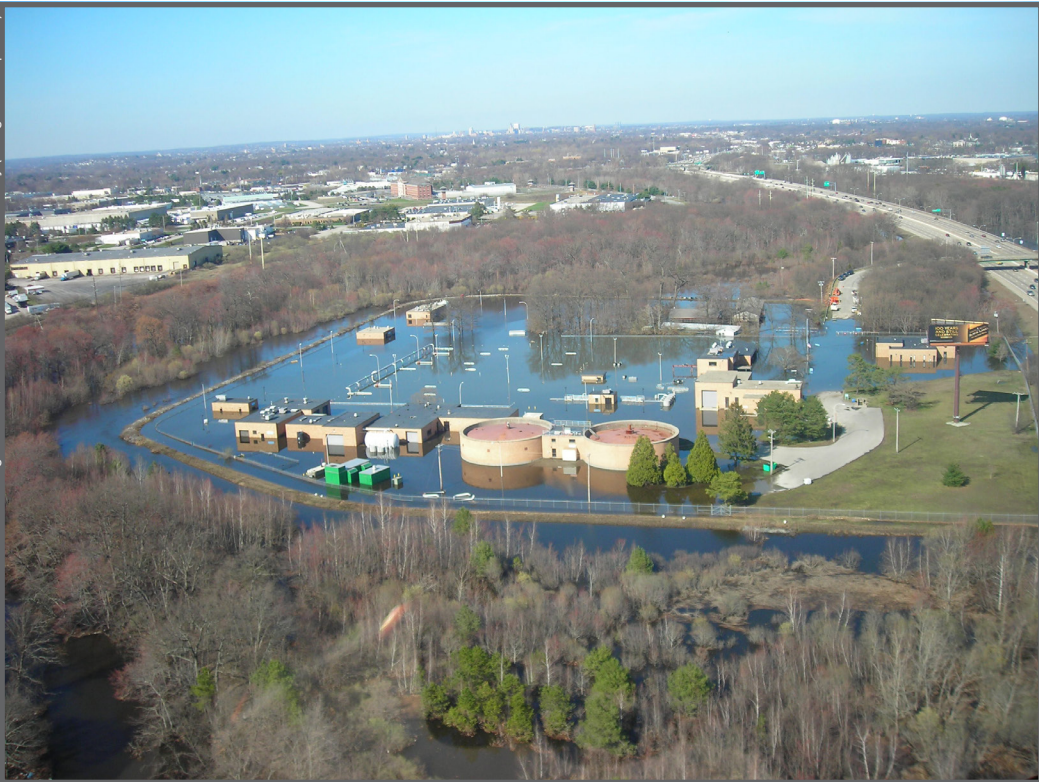
Warwick, Rhode Island Treatment Facility Flooding, 2010
