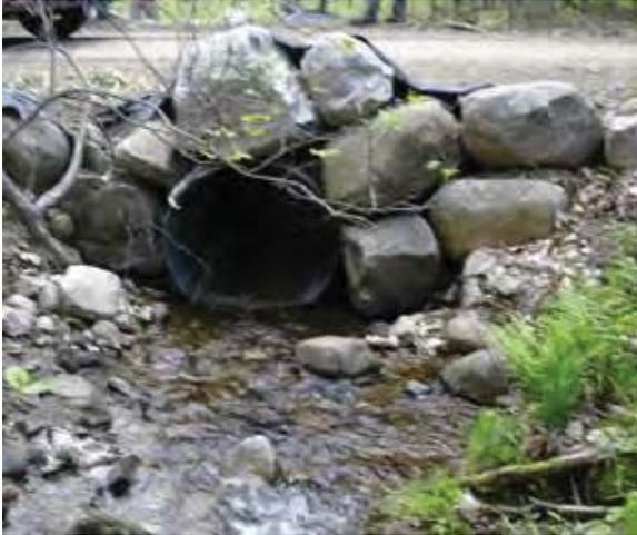
**Shallow Crossings:** Water depths are too low for many organisms to move through, and the bottom may lack appropriate stream bed material.
