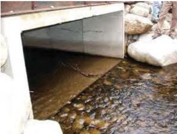
**Double Culverts:** Restriction of natural flow, clogging with debris, ponding and flooding.
