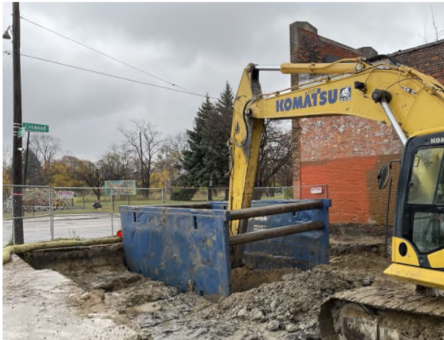
Figure 3. Contaminated soil being removed from an abandoned gas station using a trench box.
