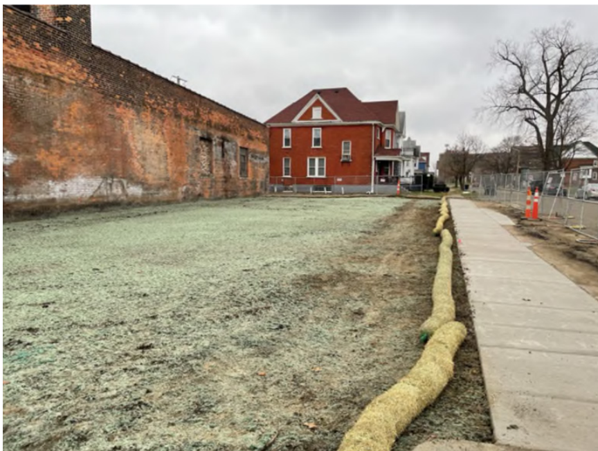
Figure 2. An abandoned gas station after being restored with topsoil and hydroseed (2024).
