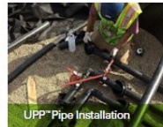
UPP™ Pipe Installation
