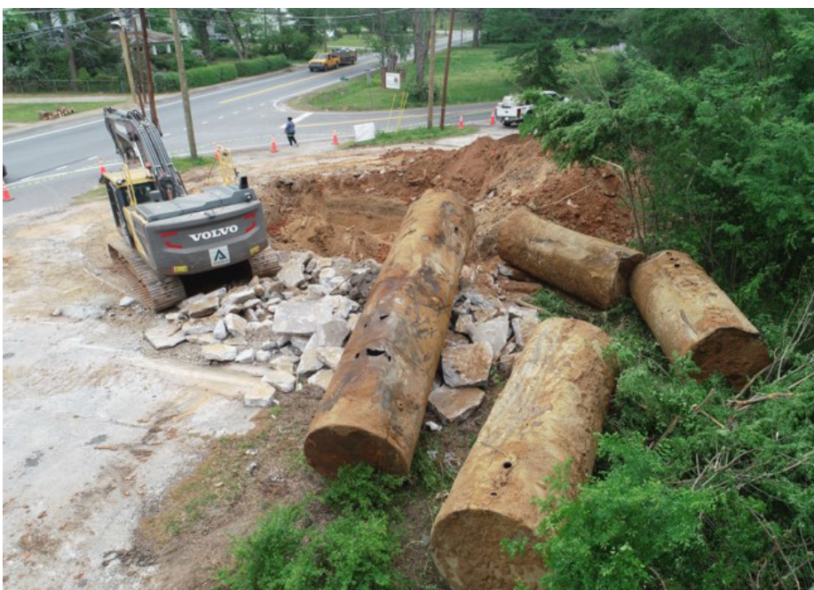
Figure 3. Tanks that have been removed from a site in Woodruff.
