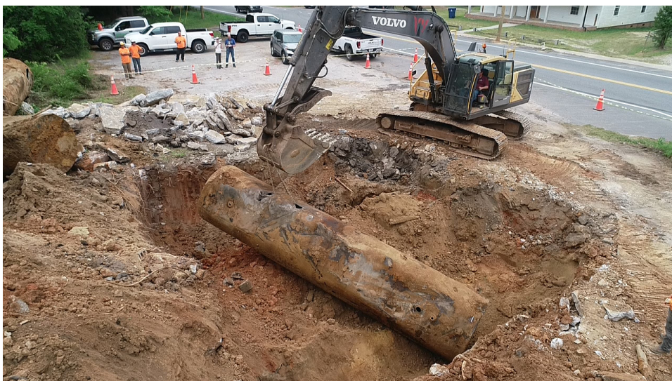
Figure 2. Click the image to view a drone video showing the process of a tank removal in Woodruff.
