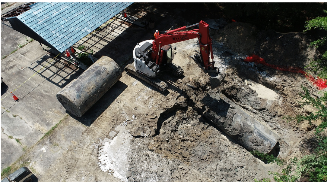
Figure 4. Click the image to view a drone video showing a tank being removed in Colombia, South Carolina.
