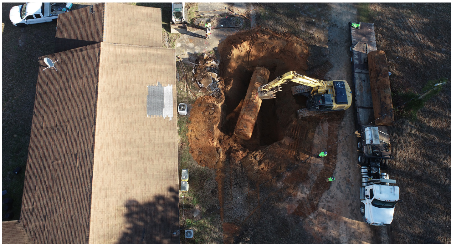
Figure 1. An aerial shot overlooking an UST removal for site 19247 in Eastover.
