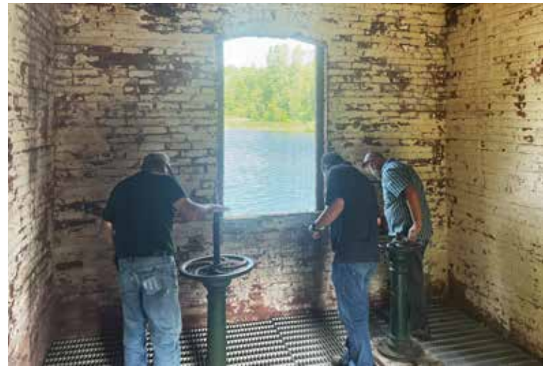
Exploring the pumphouse at the Patterson Reservoir in Plattsburgh, New York, a system that was built in the early 1900s.
