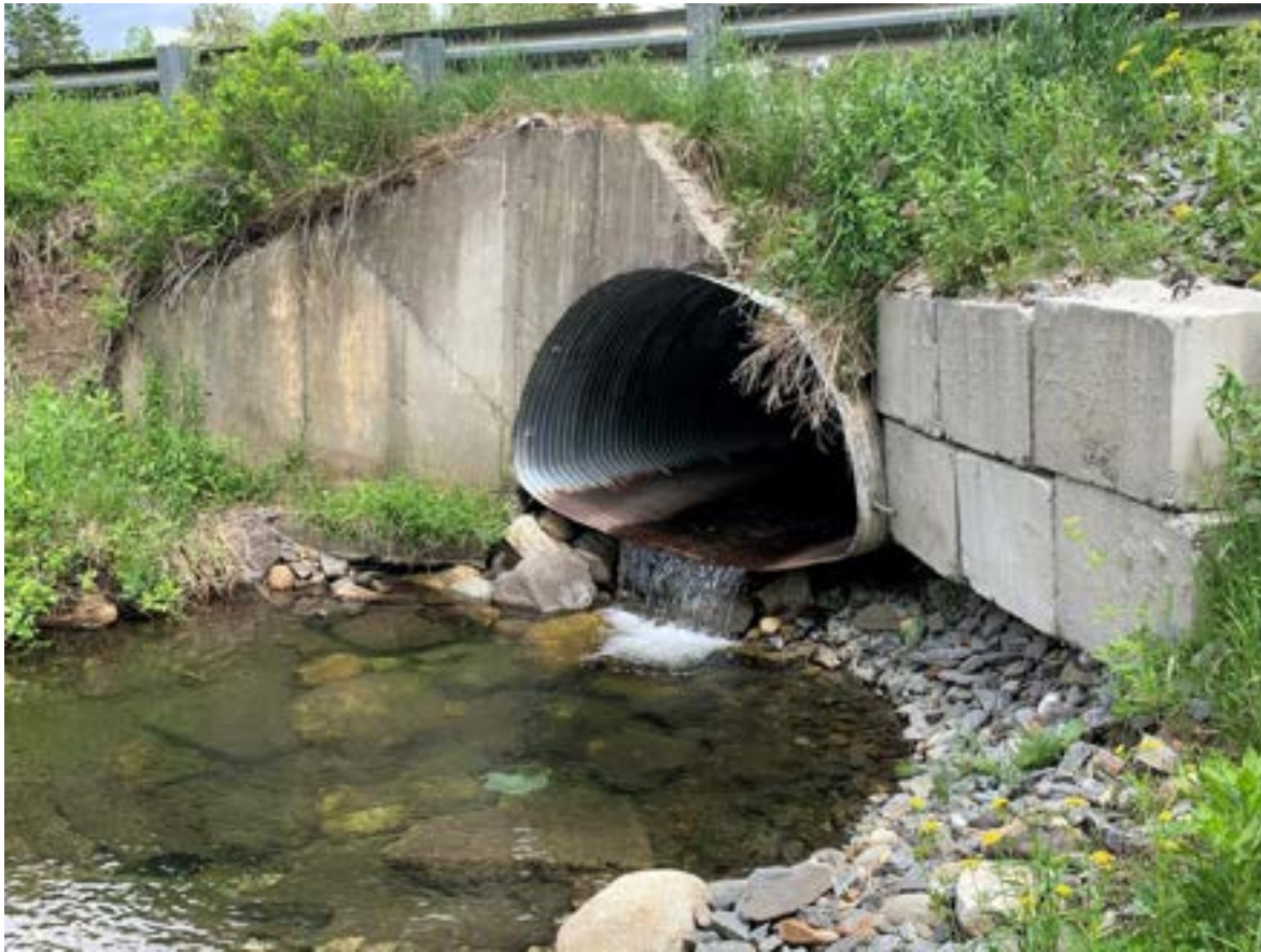
Figure 1 Hutchins Farm Rd culvert before construction
