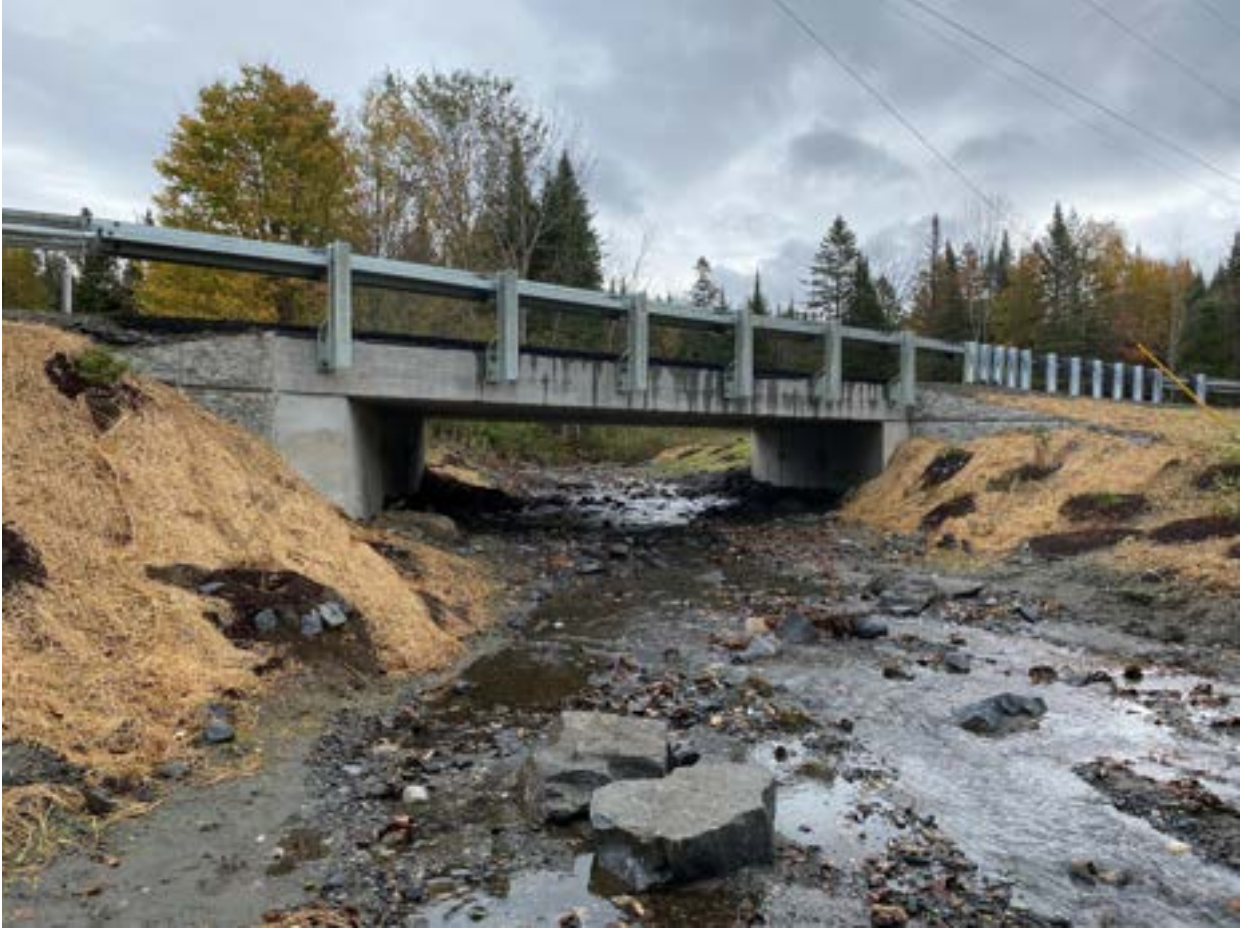
Figure 2 Hutchins Farm Rd bridge after construction
