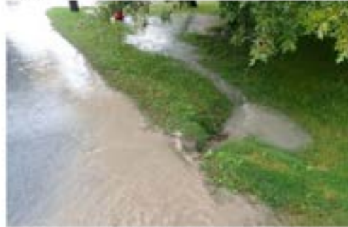
Flooding and Storm Inlet at 75 Elm Street
