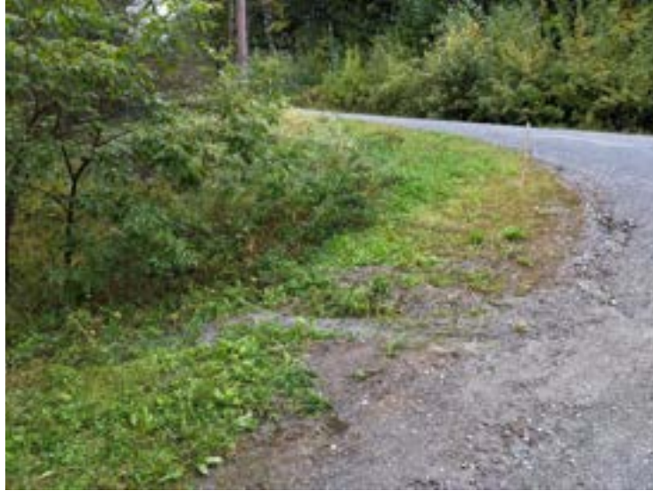
Figure 4. Black Woods Road before work was completed.
