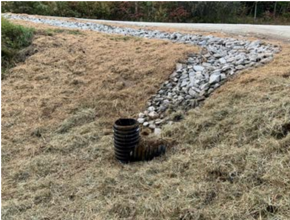
Figure 6. Black Woods Road recently after construction was completed.
