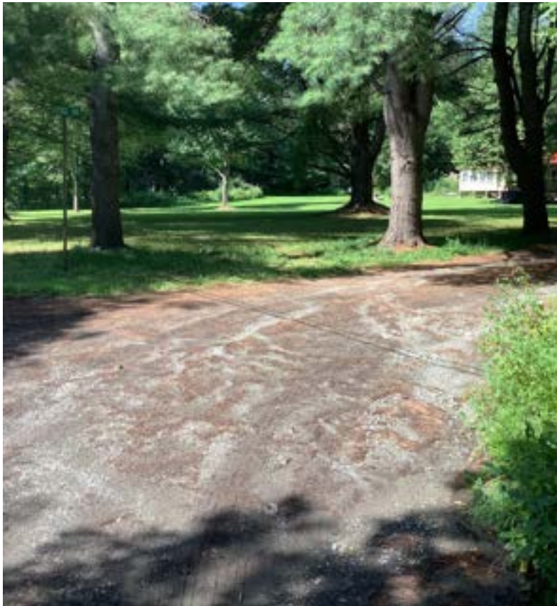
Figure 5. Existing conditions of the intersection of Patton Shore and Ledge Drive.
