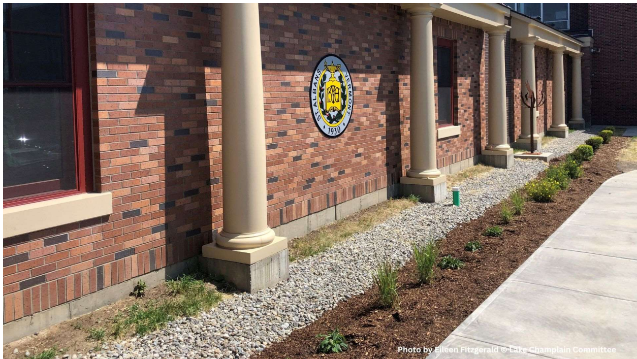
Figure 2 - The infiltration trench on the southwest side of the Connector. This section of trench is 88 feet long, running the length of the Connector under the roof's dripline. It is filled to a depth of 30 inches with washed 1" stone.
