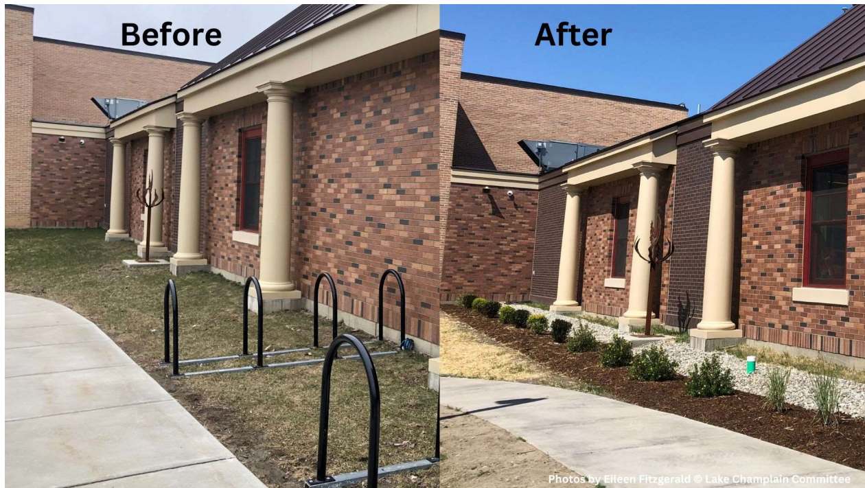
Figure 1 - The northeast side of the Connector before and after building the infiltration trench and adding native shrubs to hold soil and reduce stormwater flows. The lawn did little to retain water during rain events and most of the stormwater would runoff into the adjacent sidewalk and parking lot. With the infiltration trench and planting, stormwater will have the chance to soak into the ground.
