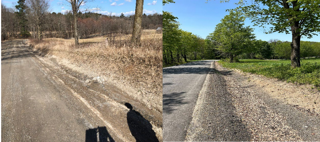
Decker Road before (left) and after implementation project (right).
