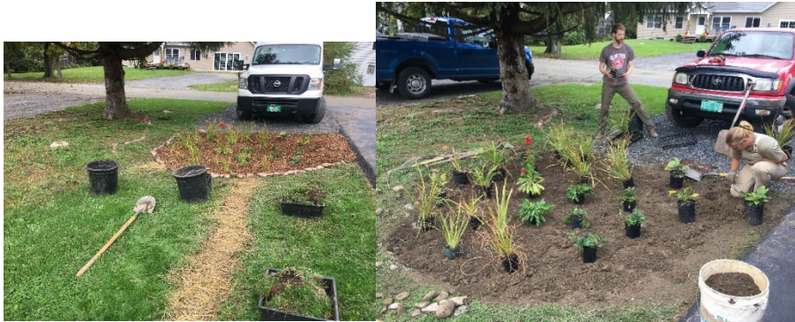
Photo 2 and 3: PMNRCD Staff installing the Johnson rain garden.
