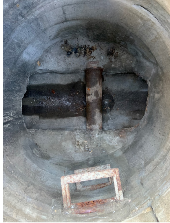
Figure 4. Sanitary sewer lateral crossing Johnson Street stormdrain
