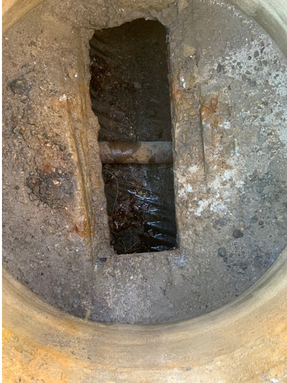
Figure 3. Sanitary sewer lateral crossing Elizabeth Street stormdrain
