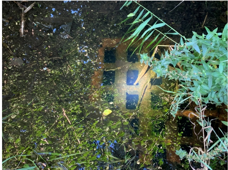
Figure 8. Flooded catchbasin CB01
