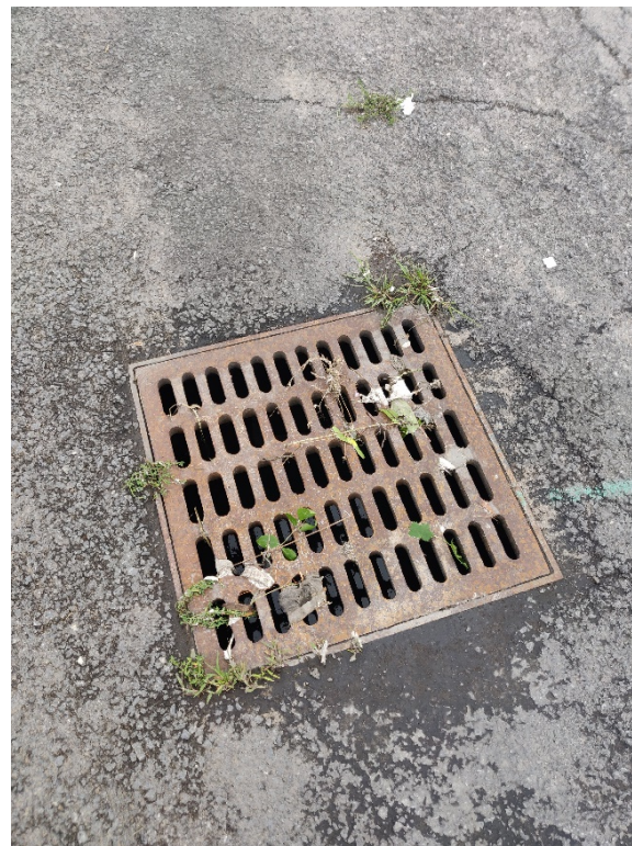
Figure 7. Toilet paper on catchbasin CB01 grate following sewer overflow event
