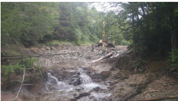
Camp Wihakowi Dam removal during construction
