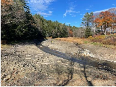
Pelletier Dam removal site post construction.
