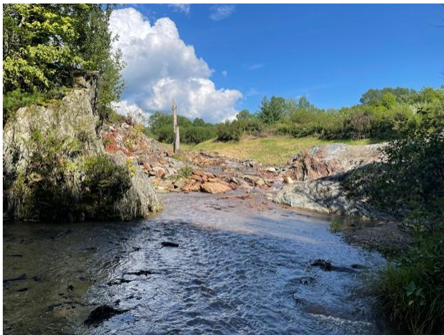
Johnsons Mill Dam post construction.
