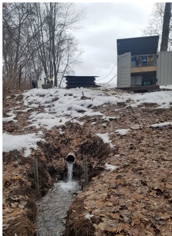
Figure 29. ACT1 tile drain outlet
