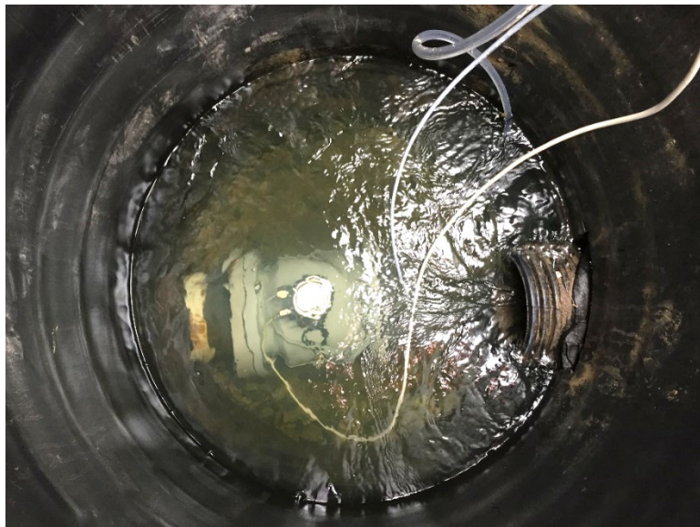
Figure 7. 8-inch Waterflux 3000 flowmeter in JBT11 manhole
