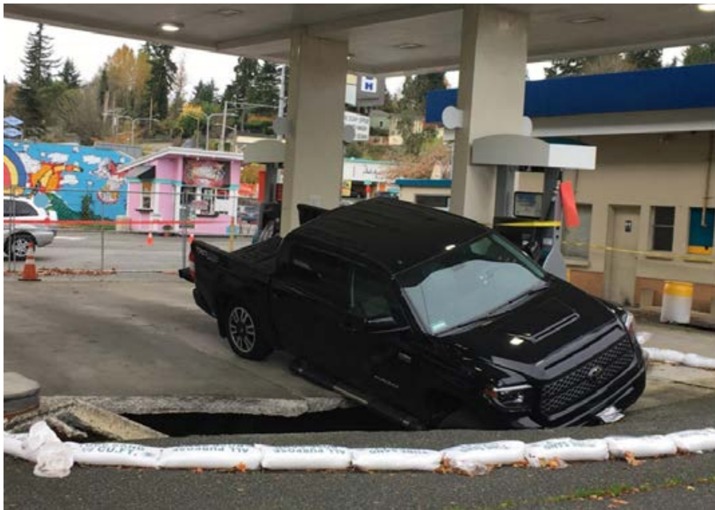
An example of cement collapse post-flood.
