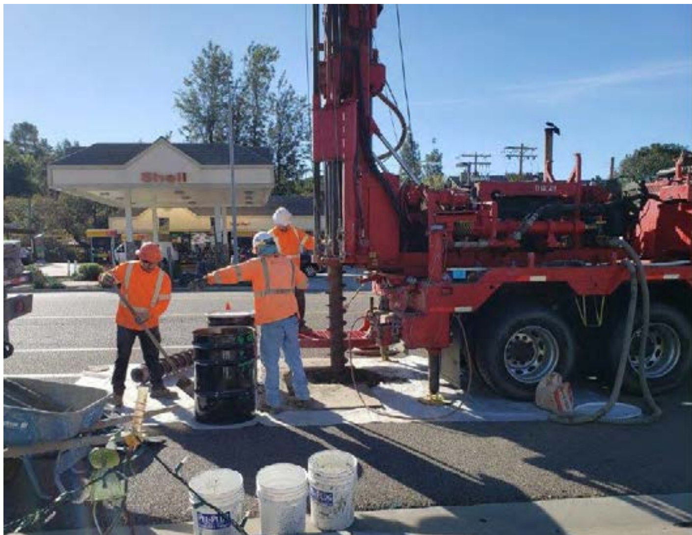
Alpine Service Station. Federal contractors properly destroying groundwater monitoring wells at a Stalled LUST Case Initiative site in Alpine, CA (October 2019). Proper destruction of site groundwater monitoring wells is often the last step in completing a LUST cleanup. Wells left in place can serve as conduits for groundwater contamination.
