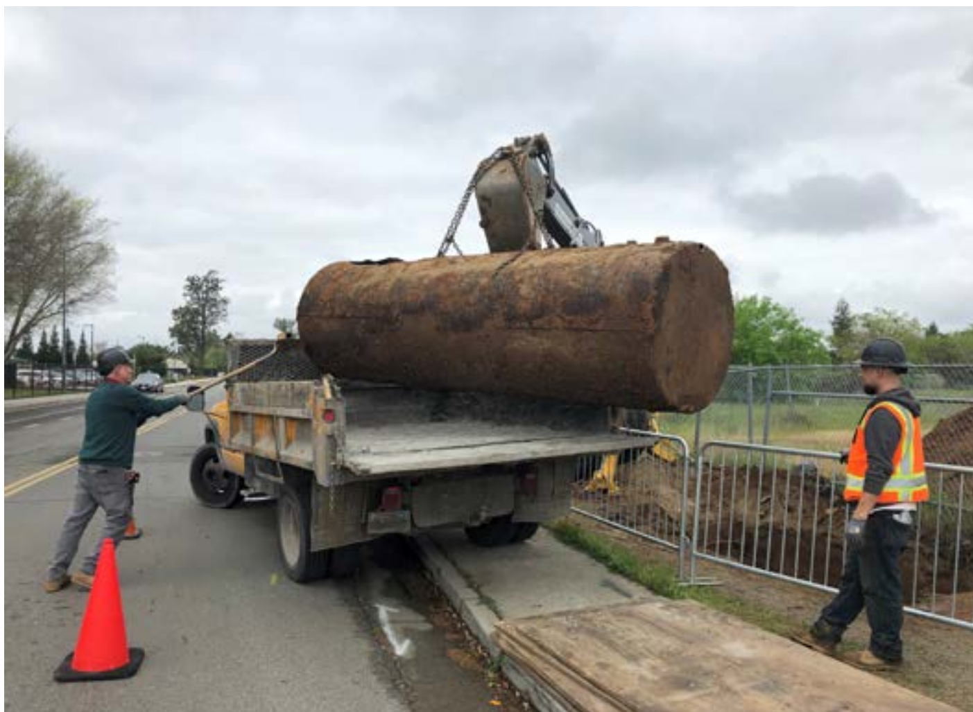
Federal contractors remove an abandoned UST as part of a two-step site assessment (January 2020) in Olivehurst, CA, across the street from Ella Elementary School. The work resulted in LUST cleanup complete.
