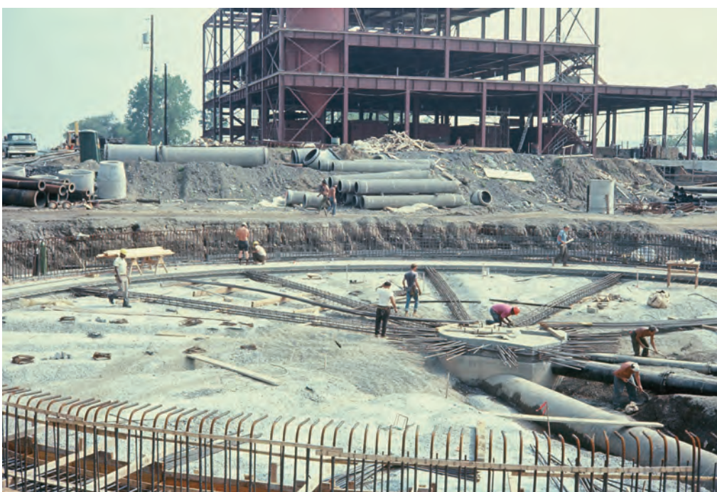
Final clarifier and solids building, North Plant.
