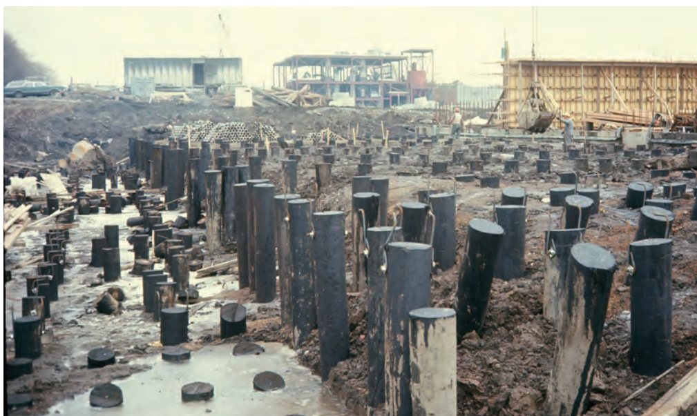
Timber pilings, South Plant.
