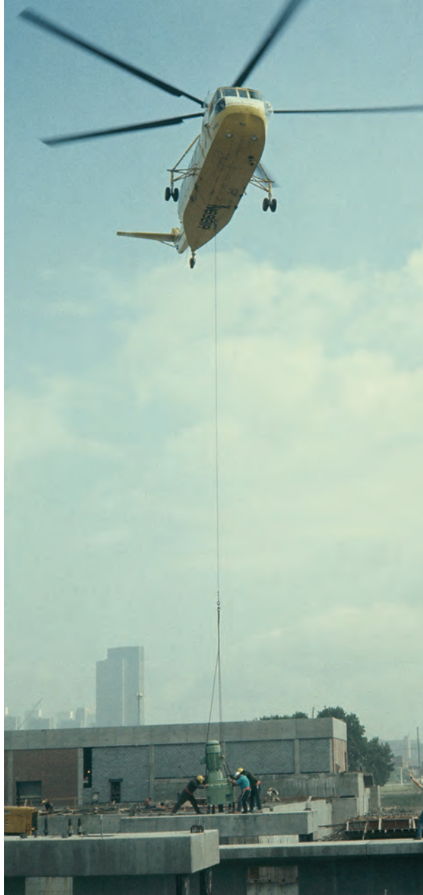
Placing the mechanical aerator motor, South Plant.
