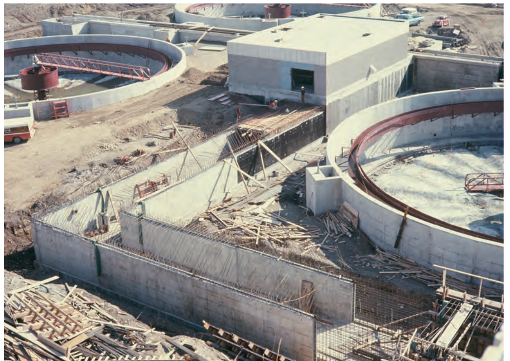
Administration building, North Plant.
