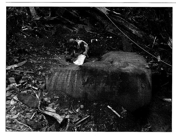
DEC inspector on top of a 20,000 gallon tank that was crushed by the partial collapse of a building.
