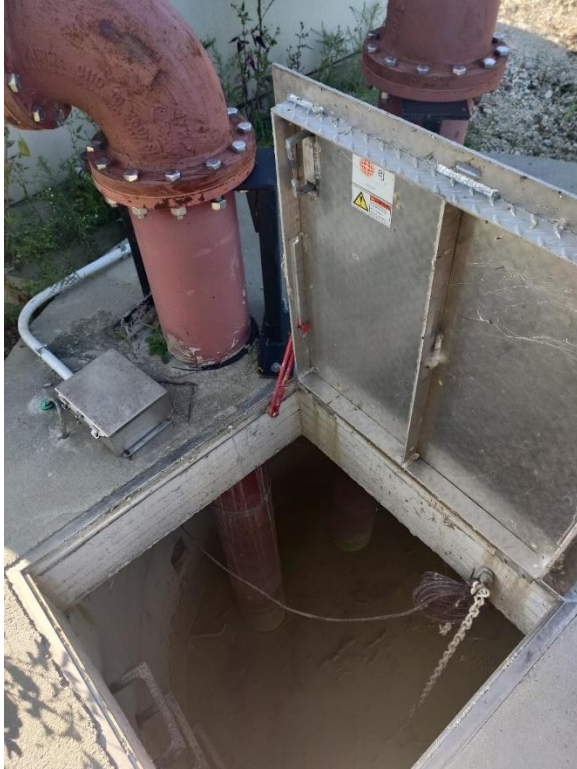
Figure 7. Suction pipes within intake vault
