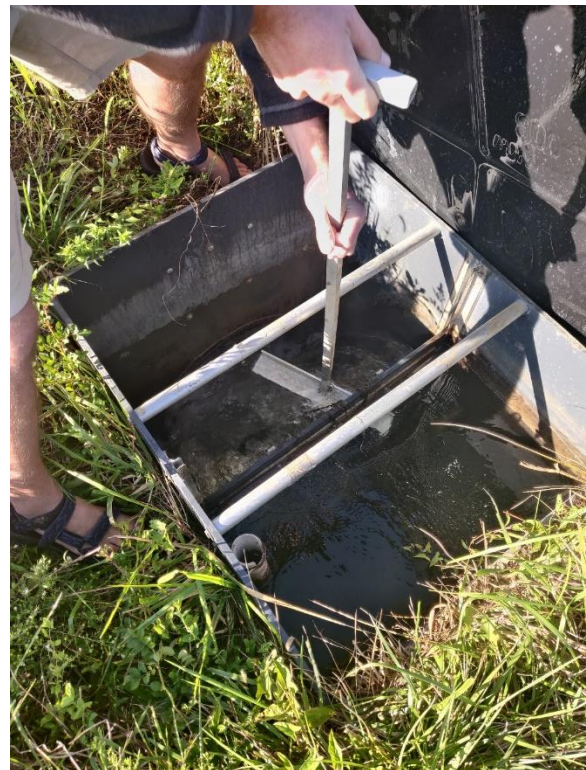
Figure 15. Adjusting stoplogs in water level control structure
