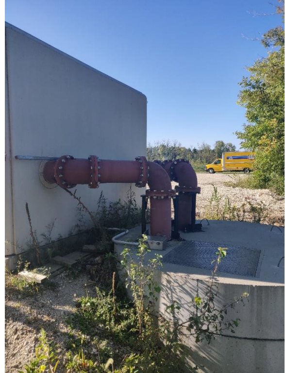
Figure 8. Suction pipe connection to vault
