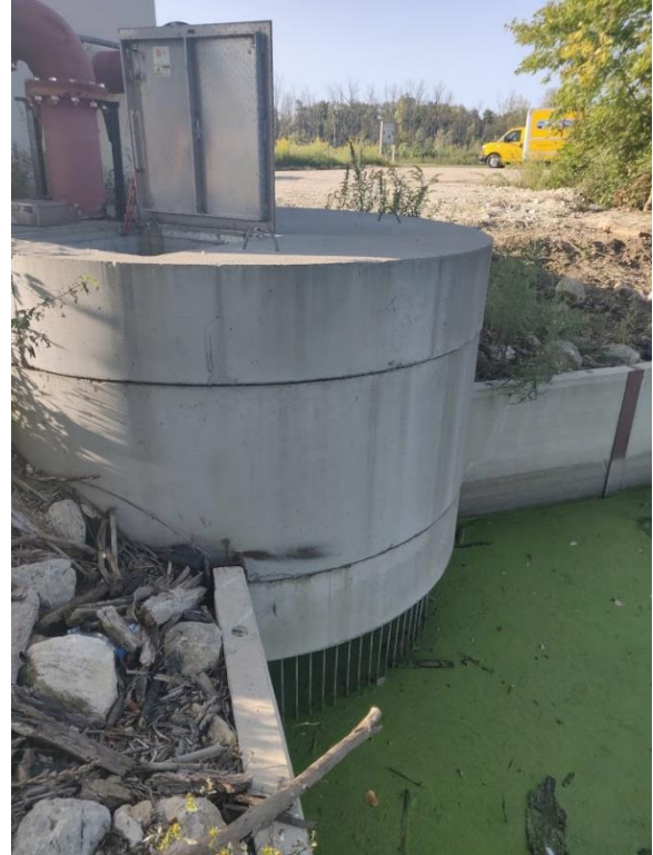
Figure 6. Intake grate
