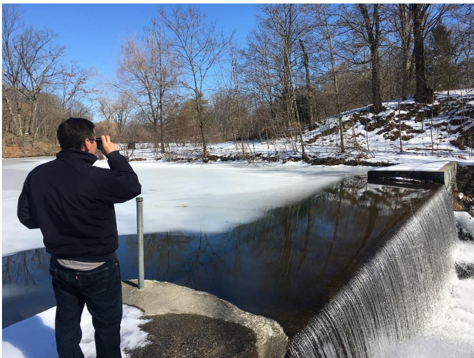
Dan estimates distances to characterize the dam as part of the “Hydrologic Conditions” portion of the assessment protocol.
