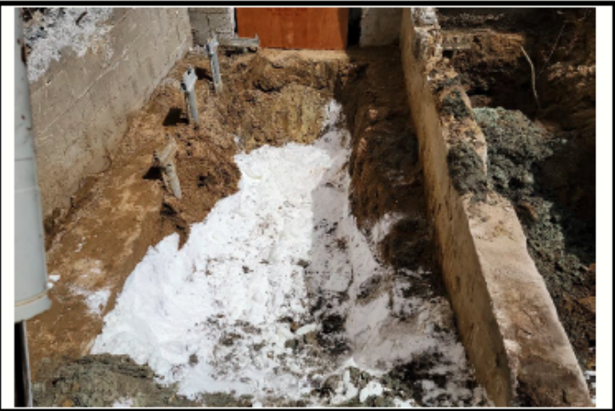
Sodium persulfate mixed with gravel was added to the excavation.
