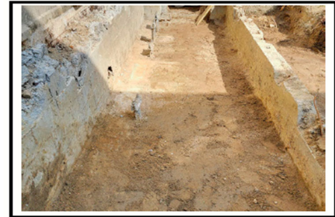
Excavation was backfilled with subsoil type S-1 (structural fill). Compaction of the backfill material occurred in approximate one-foot lifts using a vibrating compactor. Old cinderblock patio support is visible.
