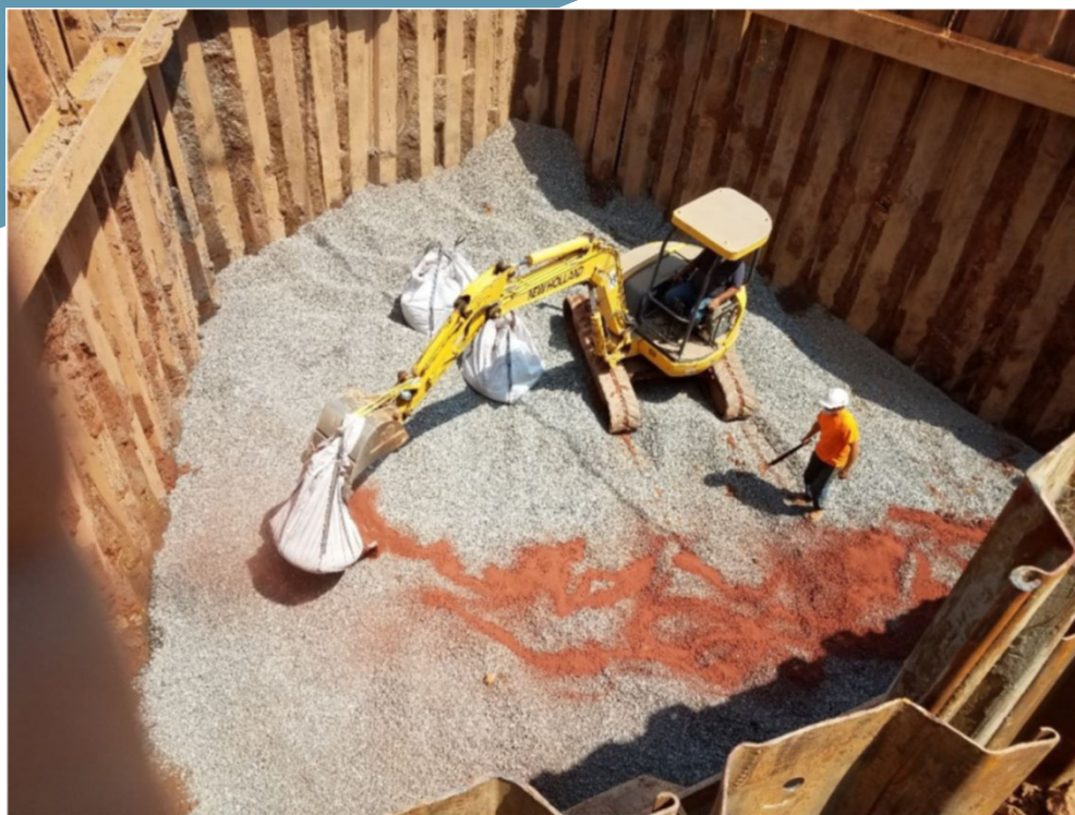
Provect-Oxs compound being distributed
