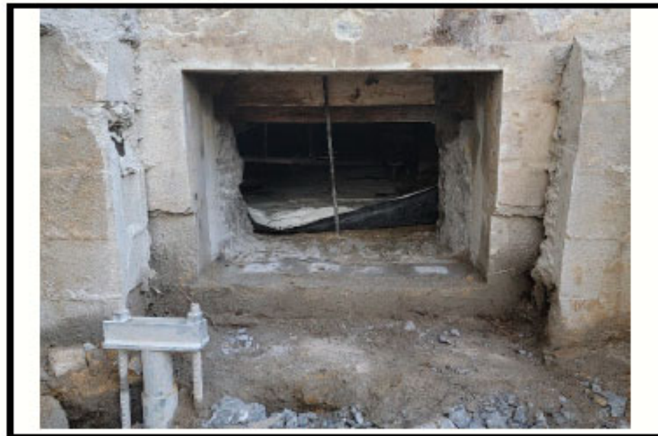
An access point to the crawlspace was installed beneath the rear entrance of the residence.
