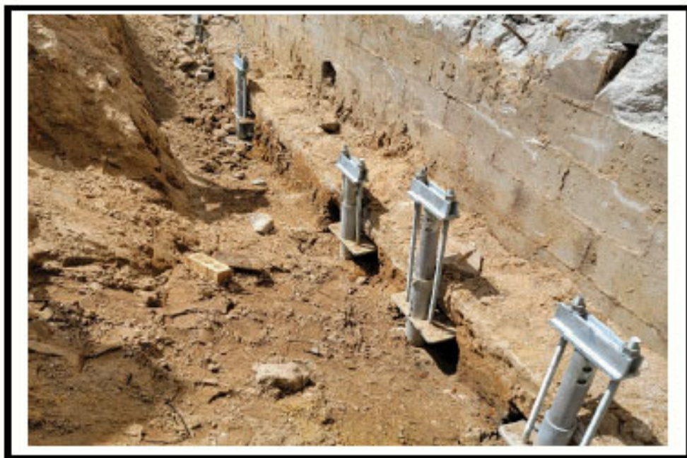
Helical anchors were installed below the concrete footings to support the residence foundation.
