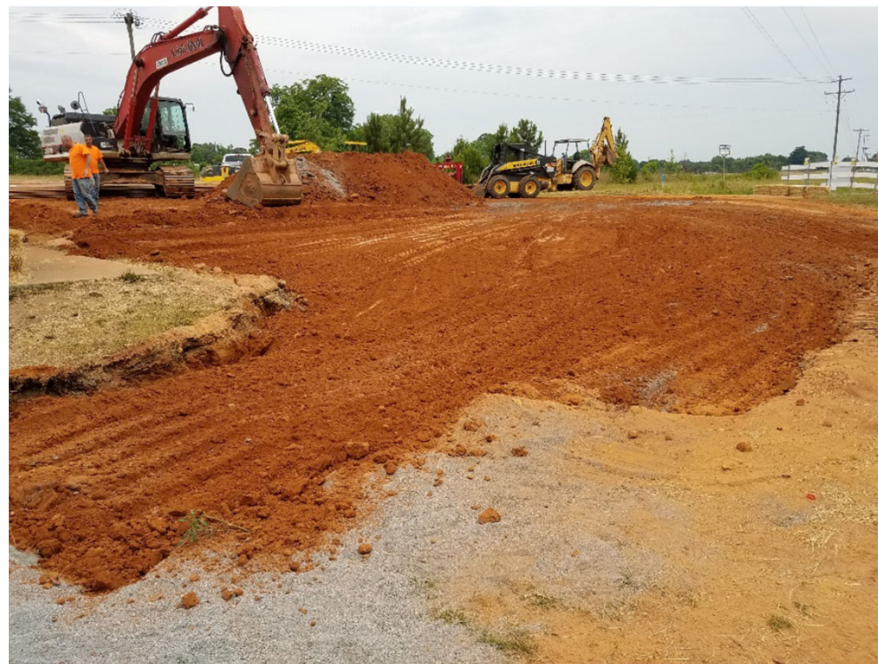
Completion of backfill and compaction
