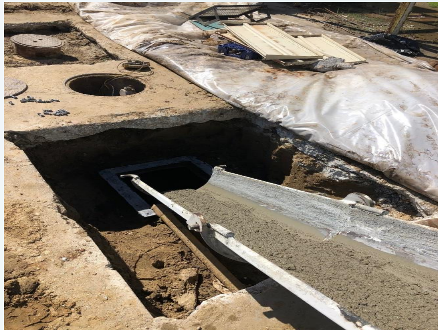
Filling with inert material
