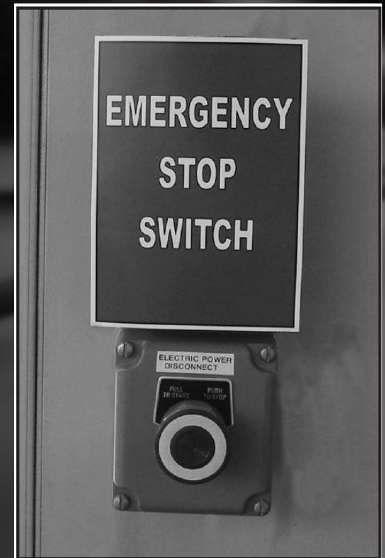
FIGURE 11-1. The E-stop should be clearly labeled and located where it is easily accessible.
