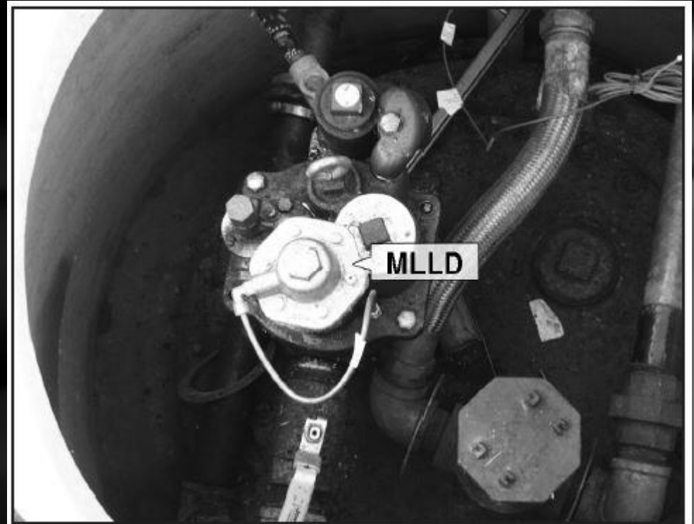
FIGURE 9-1. The MLLD mounted on the submersible turbine pump will restrict flow when a leak is detected.
