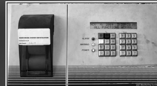
FIGURE 8-1. The indicator lights and the LCD display on the monitoring console show the status of the UST system.
