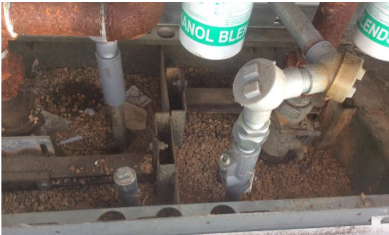
Wet spot in gravel under dispenser from fuel seep.
