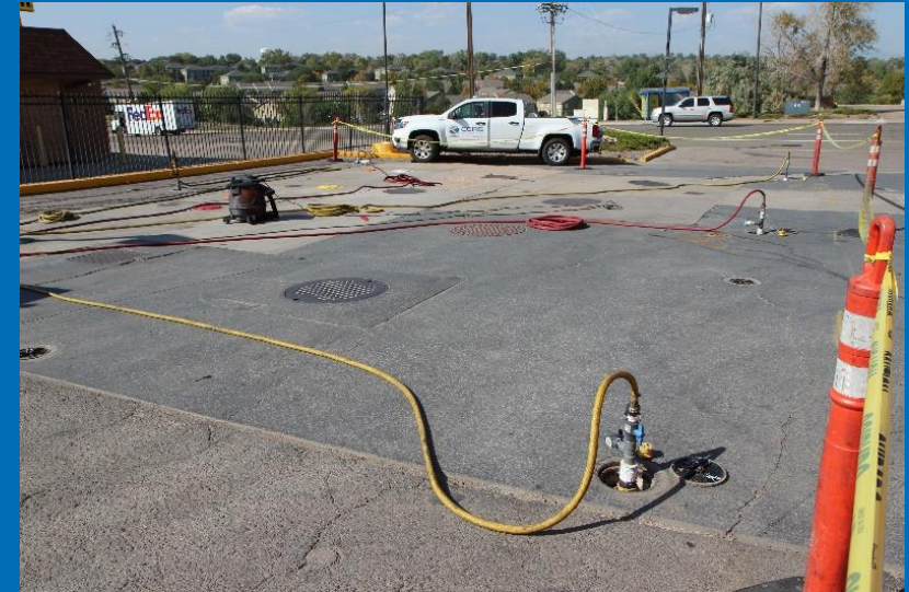
UST Basin Floods
