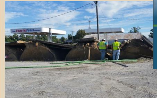
Examples of USTs affected by buoyancy. Hurricane Matthew, 2016. Credit: NCDEQ
