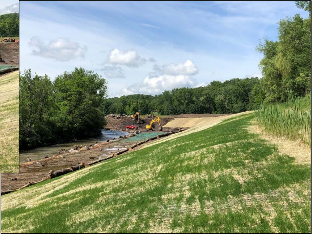
Root wad placement and floodplain construction
