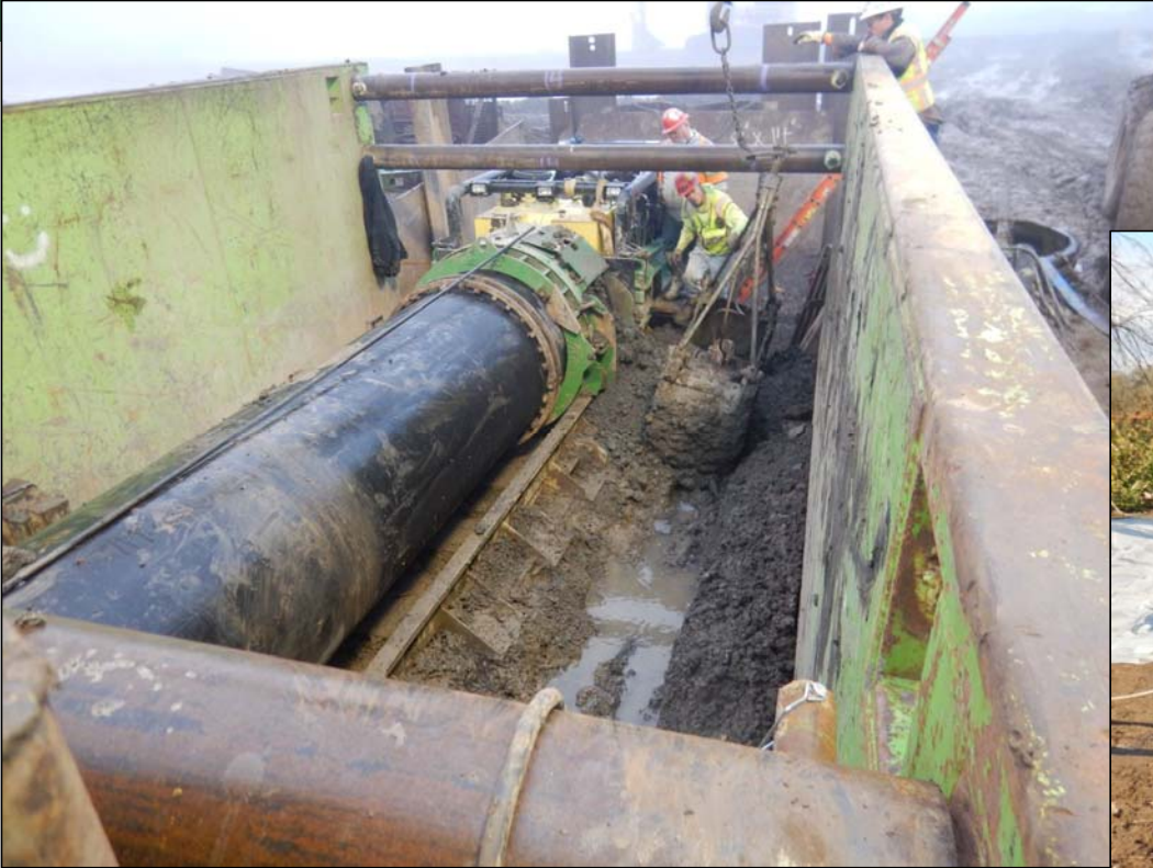
Jack and bore new 48" culverts under CSX railway
