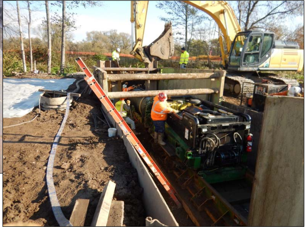
Jack and bore new 48" culverts under CSX railway
