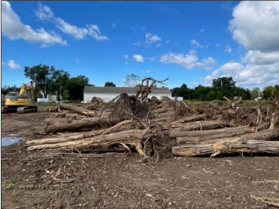
Root balls ready for installation
