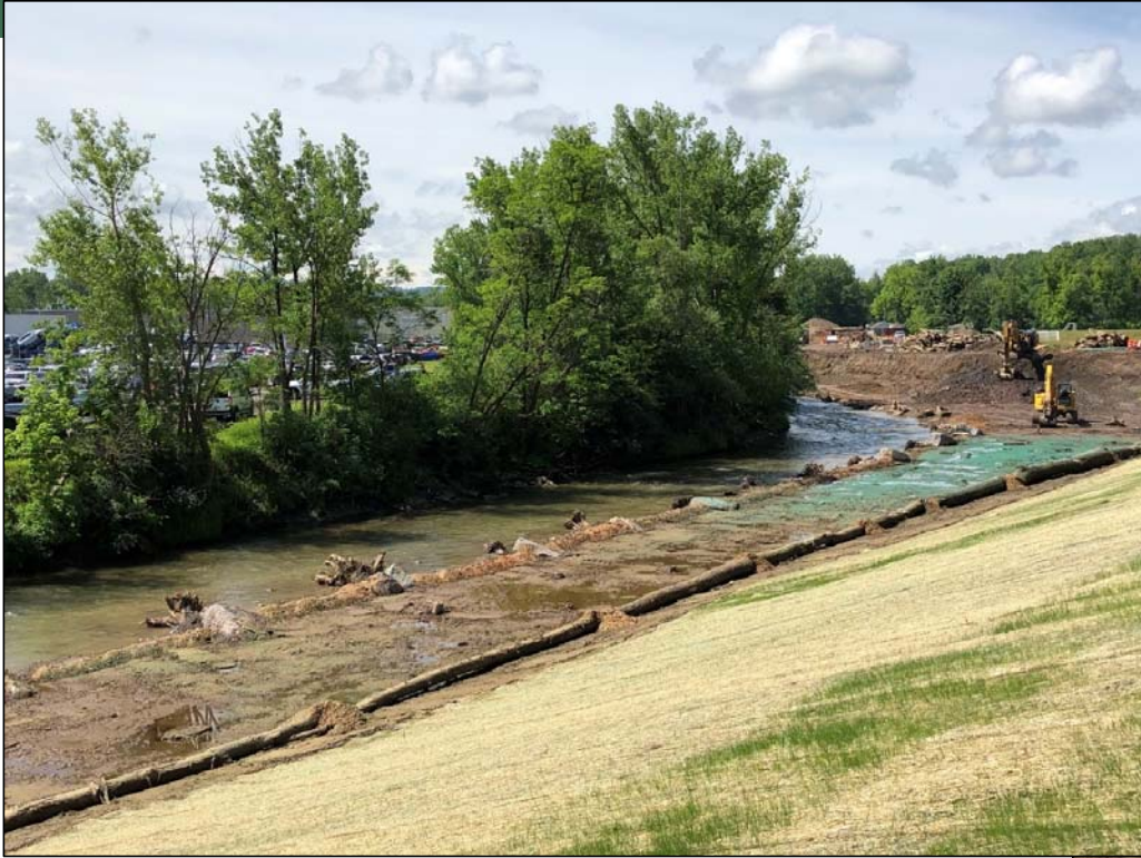
Root wad placement and floodplain construction
