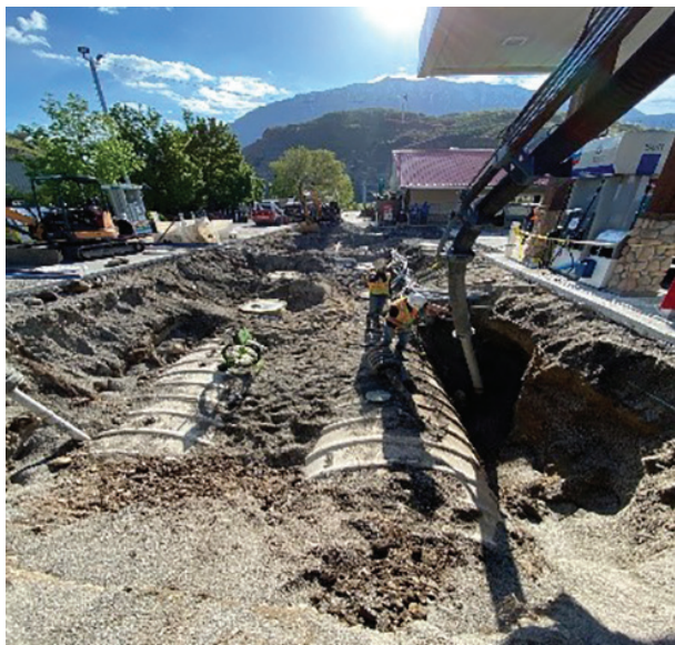
Figure 1 View of the pea gravel fill being removed by a vacuum truck.
