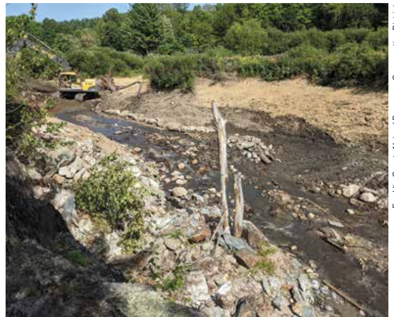
Streambank stabilization along the Bogue Branch in Bakersfield, VT.
