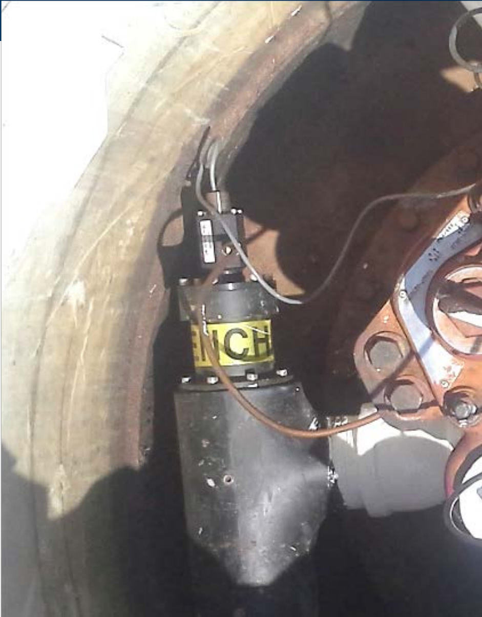
VMI LLD with sensor at left monitors piston movement. VMI controller at right shuts down STP if LLD stays closed.
