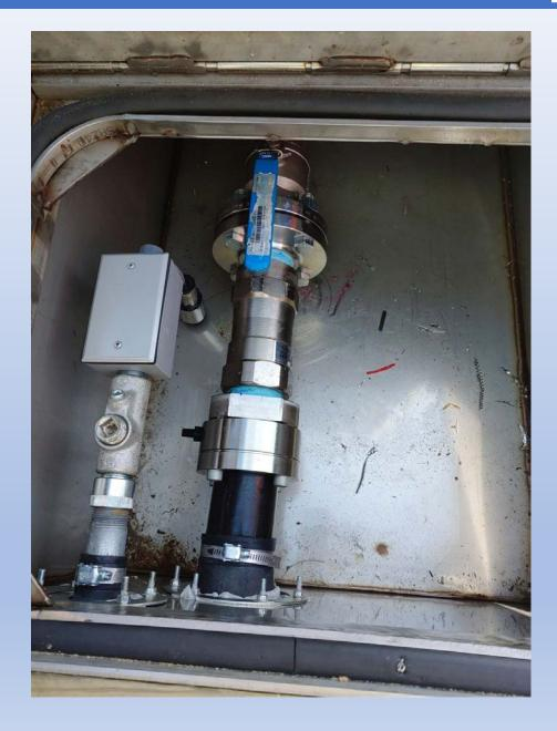
An example of a stainlesssteel dock sump with Safety Breakaway, Isolation Valve and Leak Sensor.
