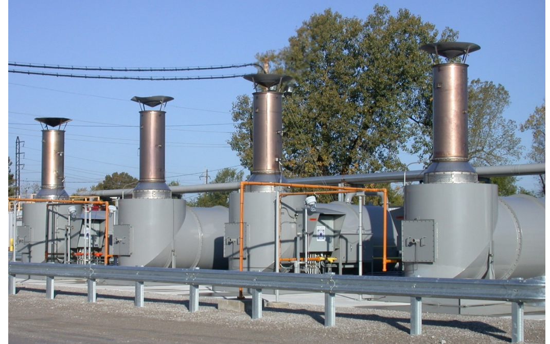
air treatment (thermal oxidizers) for soil vapor extraction (SVE) system - Hartford, Illinois
