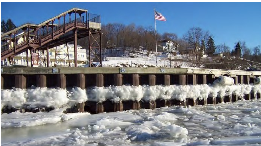
Figure 3. Rhinecliff steel sheet bulkhead at waterfront park showing ice build-up at high tide, February 2011.
