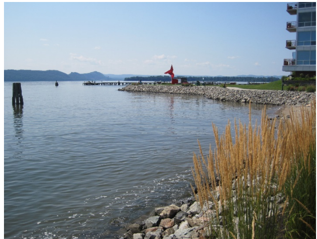
Figure . A rip rap shore edge with vegetation, foreground, and without in Ossining. (Source: DEC)
