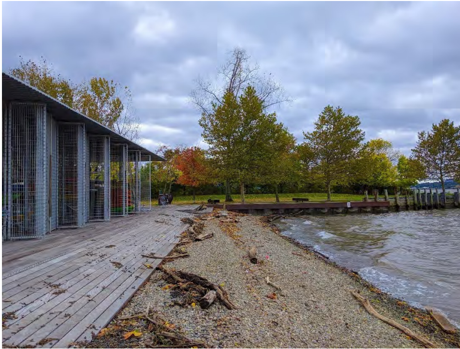
Figure 7.2 Long Dock Park features a wet floodproofed kayak shed. Note accumulation of wack and woody debris on the shore (Source: WSP)
