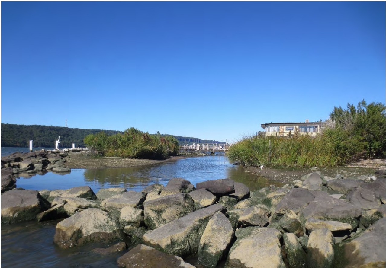
Figure 6.3 Marsh sill at Habirshaw Park, Yonkers. Rock sill protects an intertidal pool. (Source: DEC)
