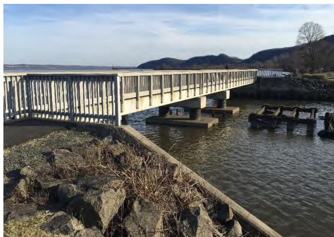
Figure 7.9 New ADA-accessible bridge features decking designed to break away, keeping the metal bridge structure in place (Source: DEC)
