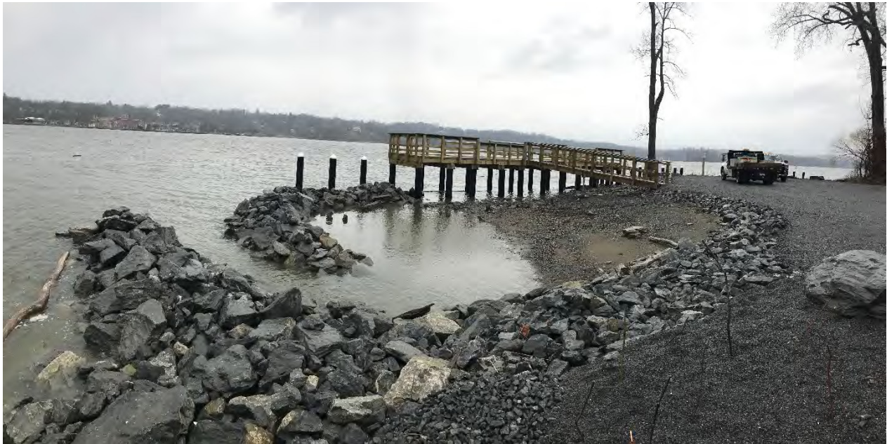
Figure 5.7 ADA accessible fishing pier. The bottom of the deck was constructed 3.1 feet above the mean higher high-water elevation, Ferry Landing at Nutten Hook, April 2020. (Source: DEC)
