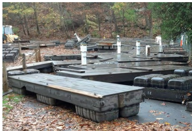
Figure 7.13 Floating docks for marina stored for season in parking lot, floated by flood because they were not anchored. (Source: OPRHP)
