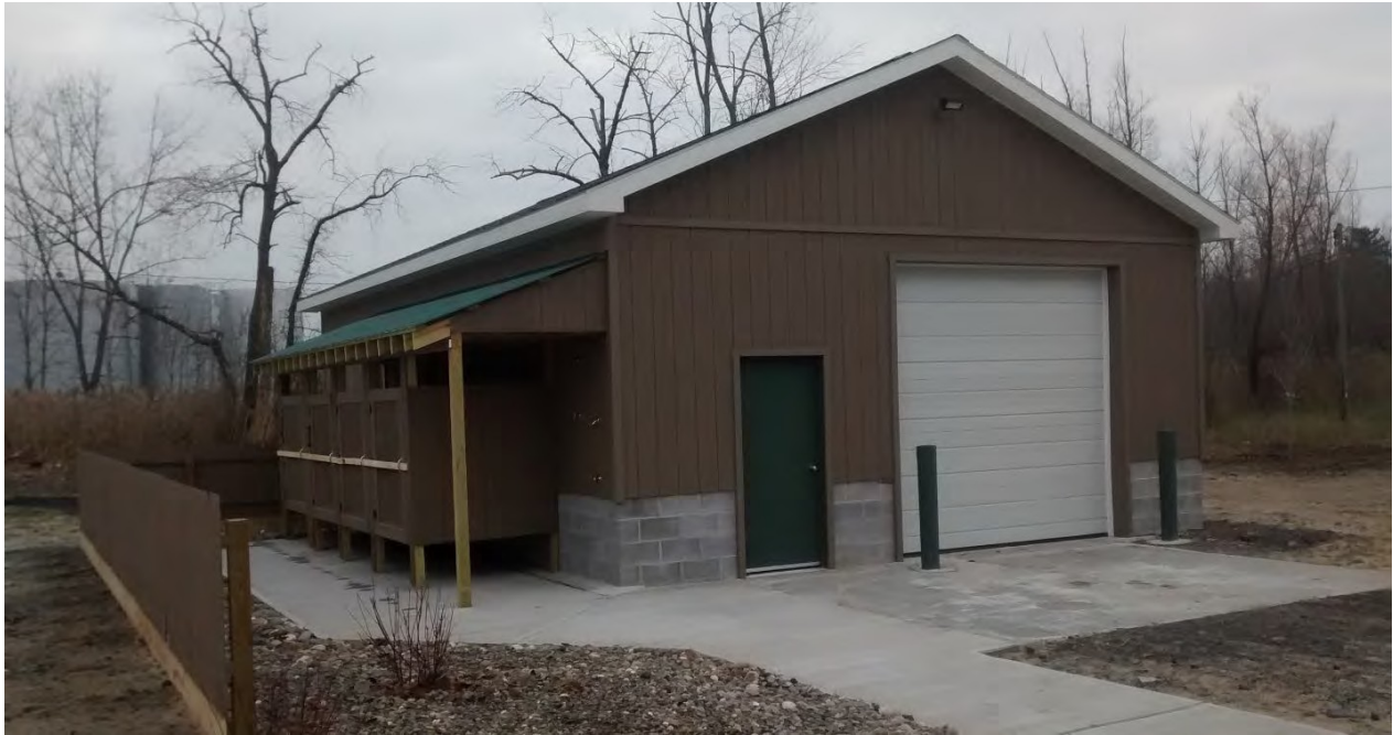
Figure 5.13 Kingston Point Park Beach utility shed showing elevated elements and wet floodproofing (Source: DEC)
