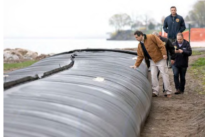
Figure 6.2 An Aqua Dam installed along Lake Ontario's shoreline in Irondequoit, NY, where severe flooding is a problem being inspected by Governor Andrew M. Cuomo (Source: Mike Groll/ Office of Governor Andrew M. Cuomo)
