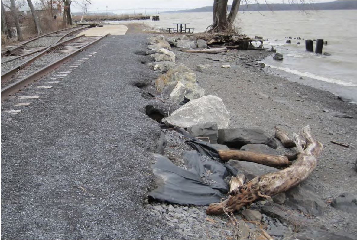
Figure 2.13 Scour along Kingston Trolley Path, April 2017 (Source: Nancy Beard/DEC)
