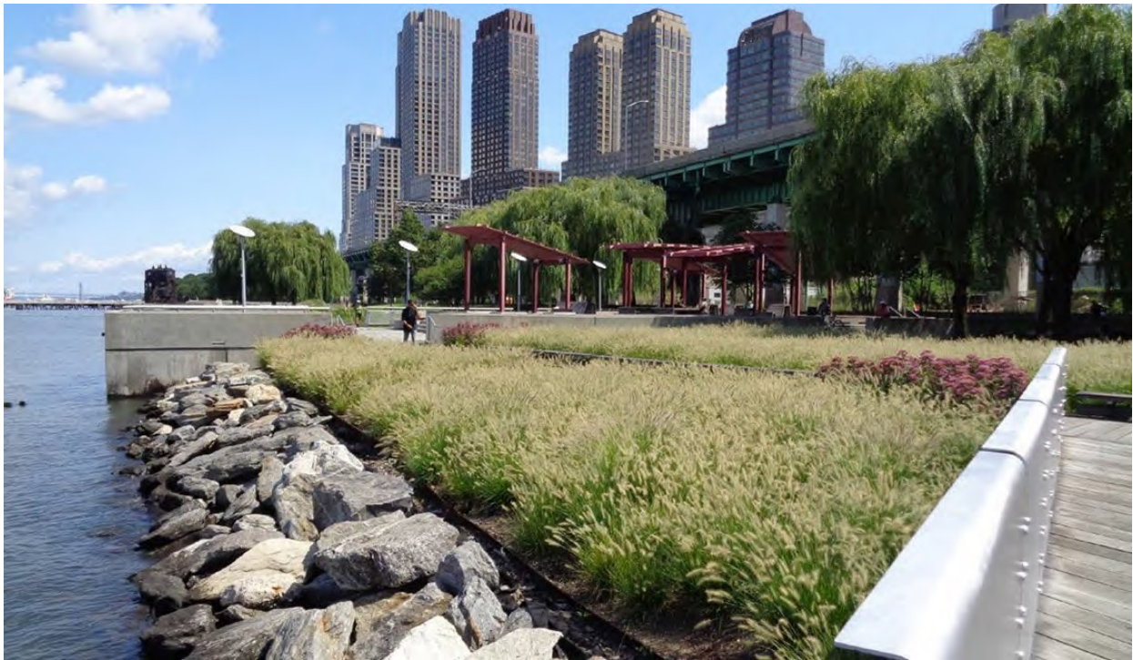
Figure 5.5 Redesigned after Superstorm Sandy, the new Riverside Park features a deeper rip rap and deeper footing in the pedestrian pathway's curb edge. (Source: NYC Parks)
