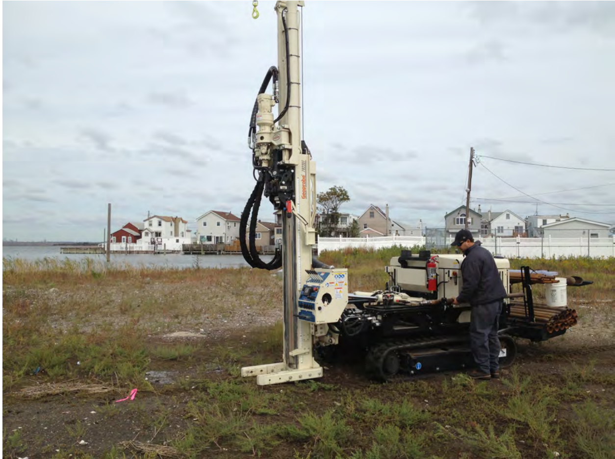
Photo 1 - Sampling using Geoprobe drill rig. View is towards the northwest.
