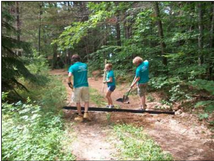
(Installing a rubber razor bar across an eroding driveway)
