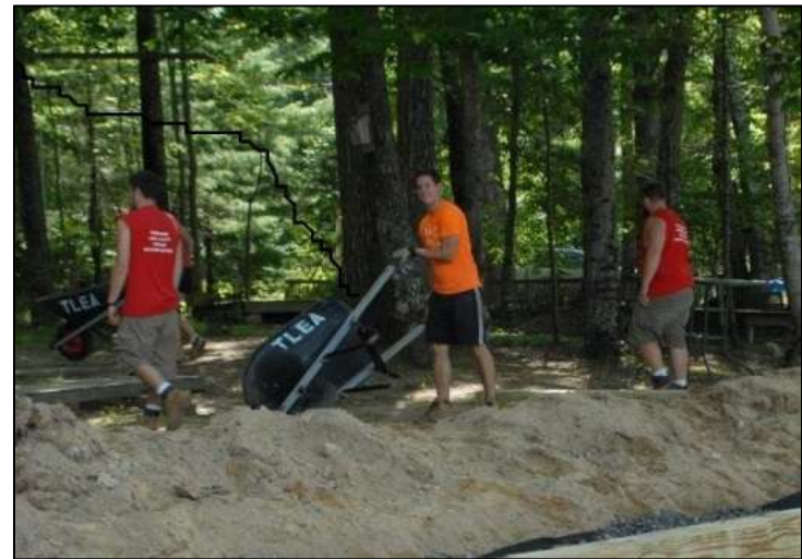
(Reinforcing a crumbling retaining wall)
