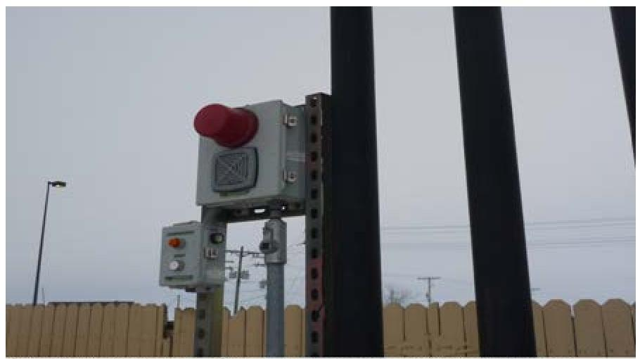
Overfill Prevention Inoperable - Confirm tank overfill alarm is properly programmed and operational for all tanks.
