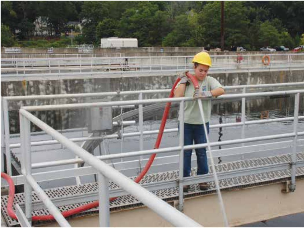
Hosing down the clarifiers at Duck Island.
