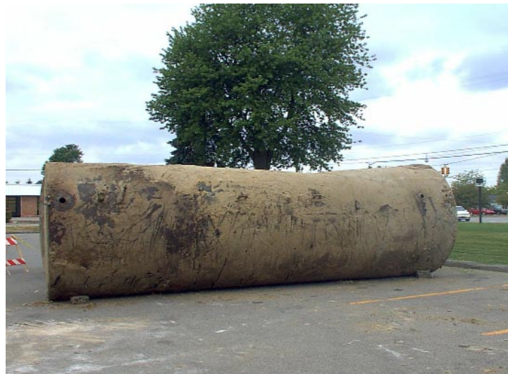
#4 Tank walls out of round
