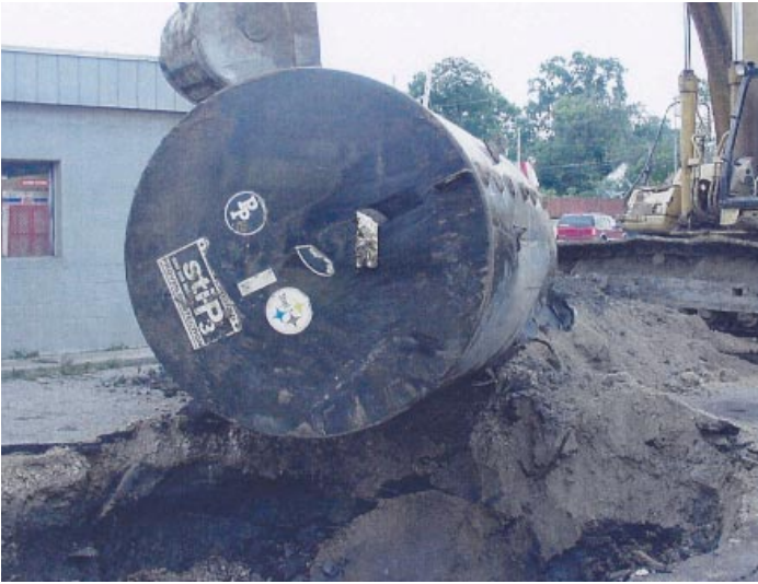
#10 STI-P3 tank in good condition.
