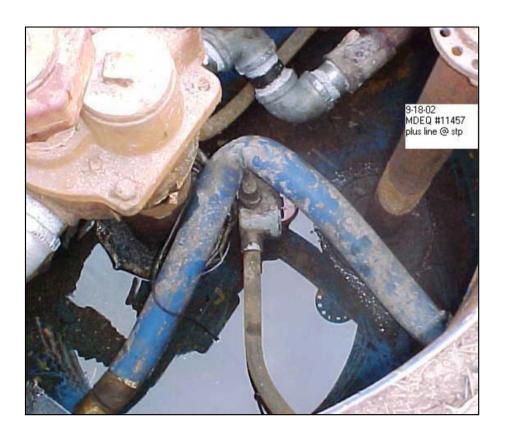
Omniflex piping also had a tendency to swell and increase in length, producing kinks that exceeded the allowable bend radius of the pipe.
