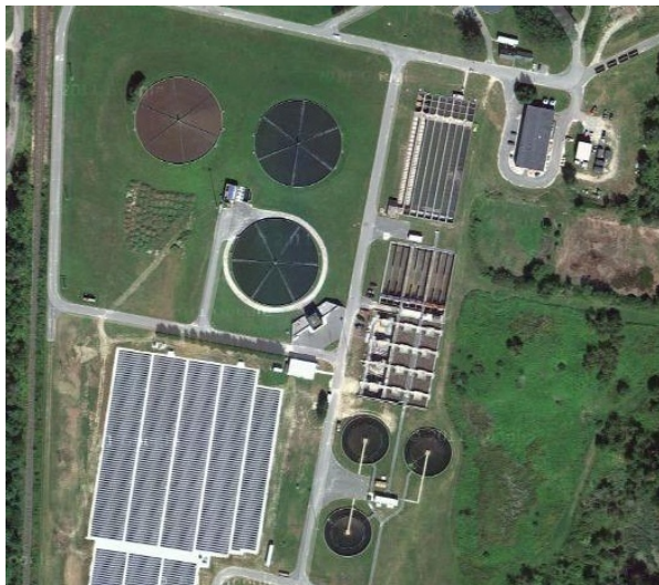
Figure PT-1 Aerial View Pittsfield, MA, Facility
