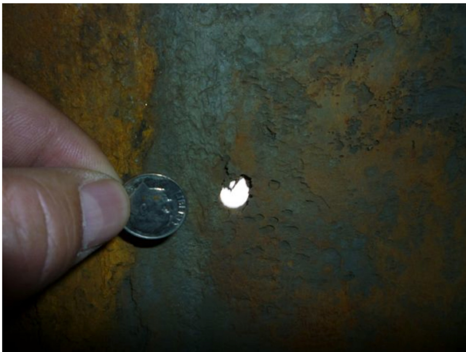
Figure 4. Internal corrosion in single-wall corrosion-protected steel tanks can produce large holes in the tank that do not leak initially because the external coating seals the hole. When the coating fails, the leak appears suddenly and the leak rate can be quite large.
