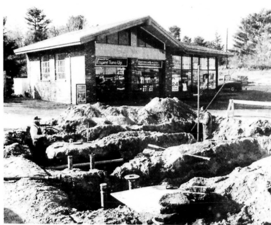
This photo from an article in The Westerly Sun, December 9, 1982, shows workmen performing tests on three USTs at the Exxon station on Route 38. Two of the tanks were leaking.
