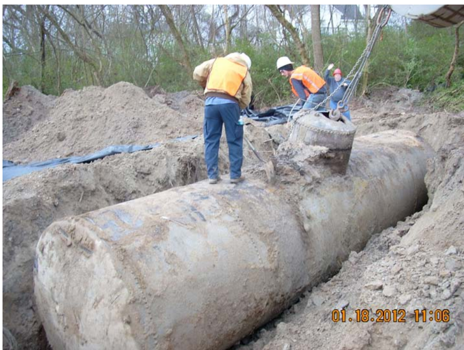
FIGURE 3. The Harrisburg Car Manufacturing Company 1888 rail car being removed from the ground. It is unknown how long this tank was buried, but there were no corrosion holes in the tank when it was excavated.
