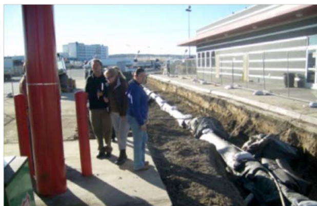
Remediation trench along diesel-fuel-release pipeline.
