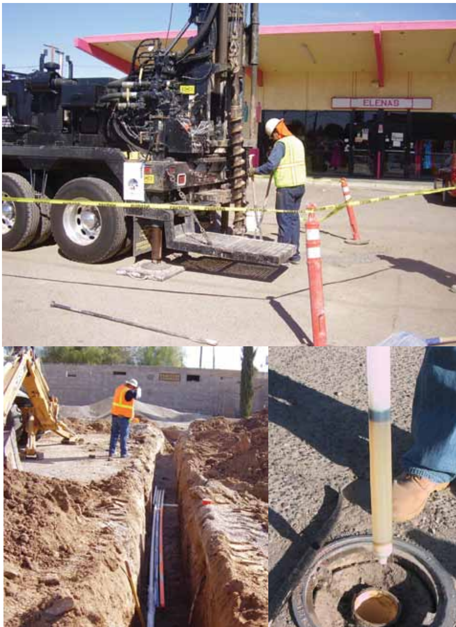
Remediation system installation and groundwater-monitoring activity.
