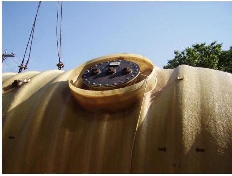
A tank equipped with a collar for attaching a full-depth sump. Such collared sumps provide secondary containment and can be used to isolate tank risers and spill buckets from the tank backfill material.
