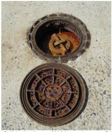
Spill bucket from a 2010 inspection at an E10 facility. Note the stalactite-type corrosion under the lid.
