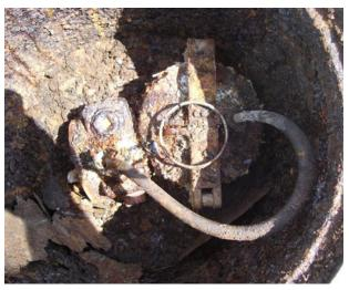
*An ATG probe area from a 2010 inspection at an E10 facility. Notice the extreme corrosion throughout.*
