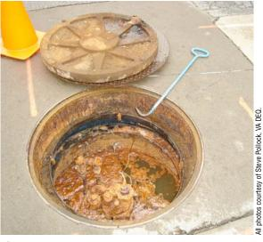
STP sump showing biological mat from a 2008 inspection at an E10 facility.
