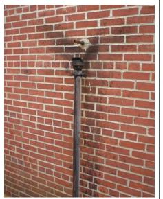
Product was released from the vent cap during an overfill event. A leak in the single-walled vent line resulting from improper installation, corrosion, or movement of the vent riser would result in a product release into the backfill during such an overfill event. Gasoline vapors and vapor condensates can also be released from these leaking vent lines
