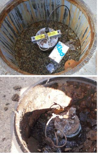
Top: Typical ATG riser installation surrounded by the tank backfill. Overfill events can leak from such unprotected risers and spill directly into the tank backfill. Such releases can be prevented by locating all risers within a collared sump.
