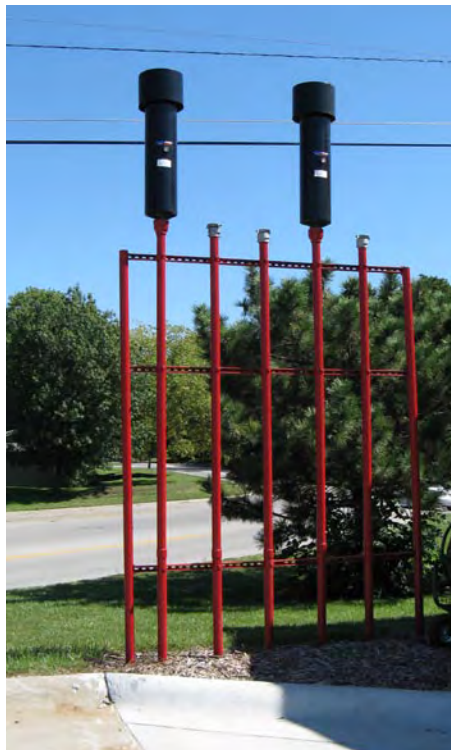
The vents for the USTs containing B-100 biodiesel and E-100 ethanol have black canisters filled with a desiccant to prevent water vapor from reaching the fuel. (Photograph: Michael L. Pomes, KDHE).
