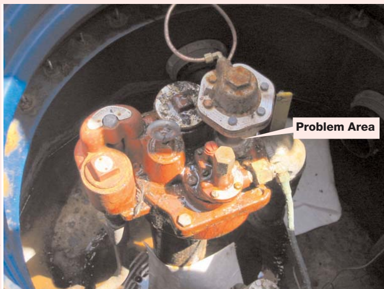
Photo: Courtesy of Marcel Moreau
