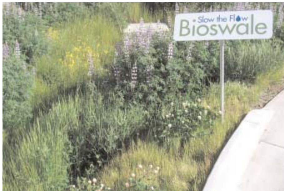
The station is bordered with grassy bioswales that contain stormwater runoff from the site, remediate contamination biologically before it leaves the site, and slow the flow of stormwater into the storm-sewer system.
