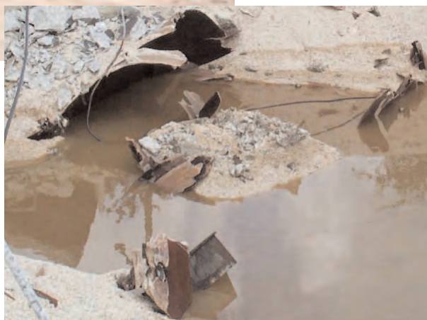
The excavation showing the remains of the diesel and premium tanks along with product. ▼
